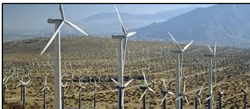
Lake Turkana Wind Power Project.
